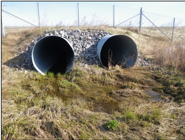
D8: Facing north (upstream) from the runningway (Spring 2015).
