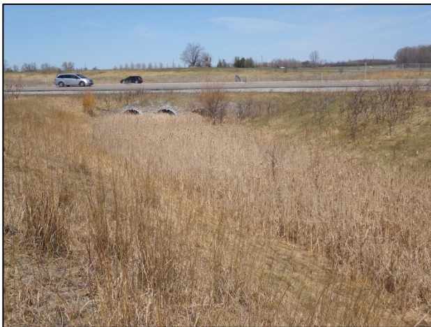
D12: Facing north (upstream) from the runningway (Spring 2015).
