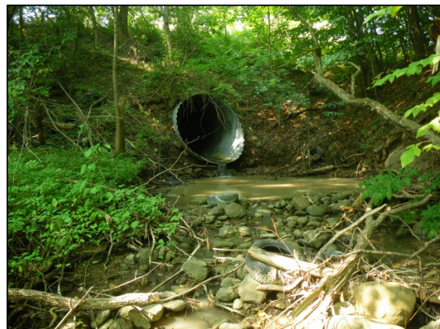
D16: Facing west (upstream) within runningway at Sideline 16 perched culvert (Summer 2015).
