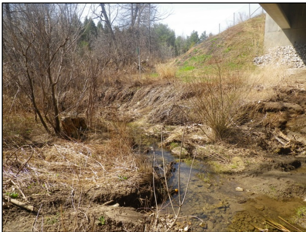
D3: Facing south (downstream) from the runningway (Spring 2015).
