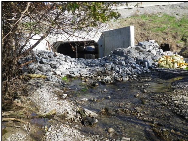
D18: Facing north (upstream) from the runningway (Spring 2015).
