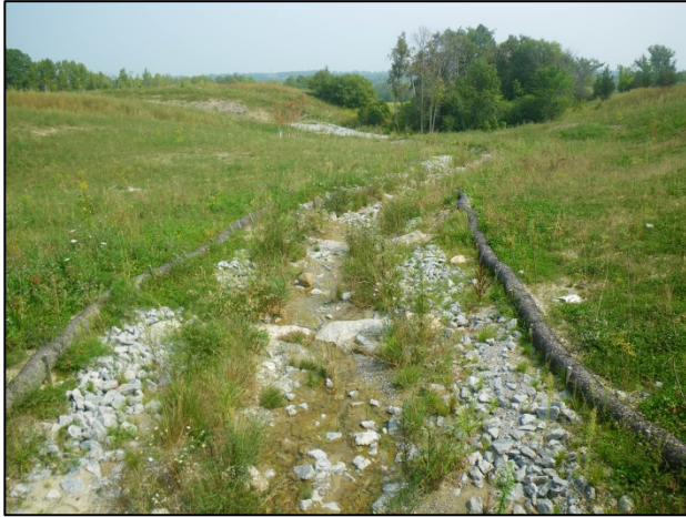
D17: Facing east (downstream) from upstream of runningway (Summer 2015).
