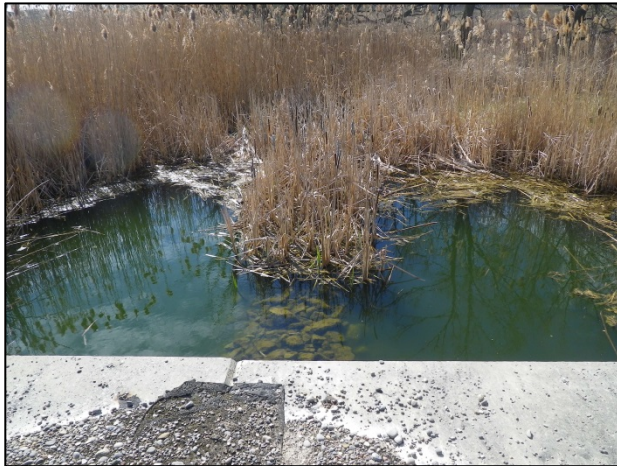
R6: Facing south (downstream) from the 407 ETR (Spring 2015).
