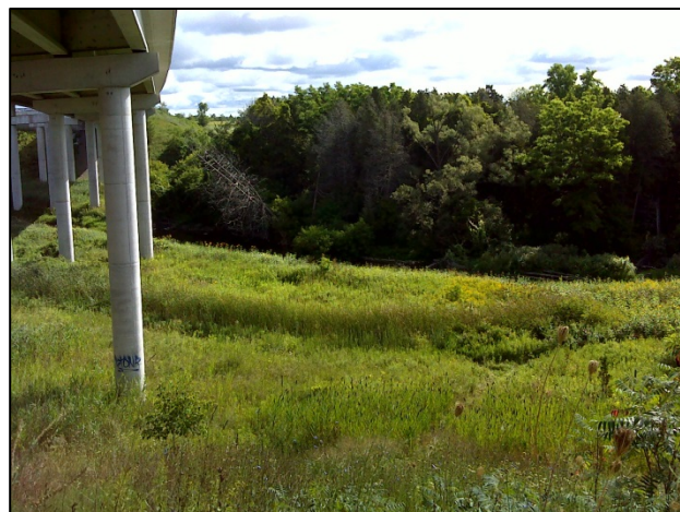
R10: Facing east, at runningway crossing (Summer 2015).
