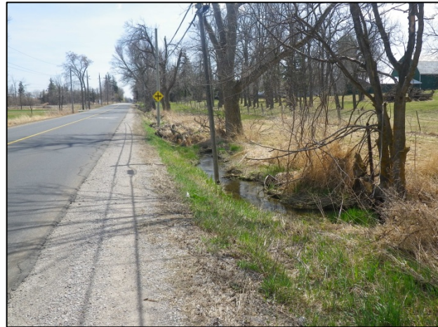
R8: Facing south (downstream) from downstream of the runningway (Spring 2015).
