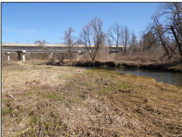
D1: Facing north (upstream) from downstream of the runningway (Spring 2015).
