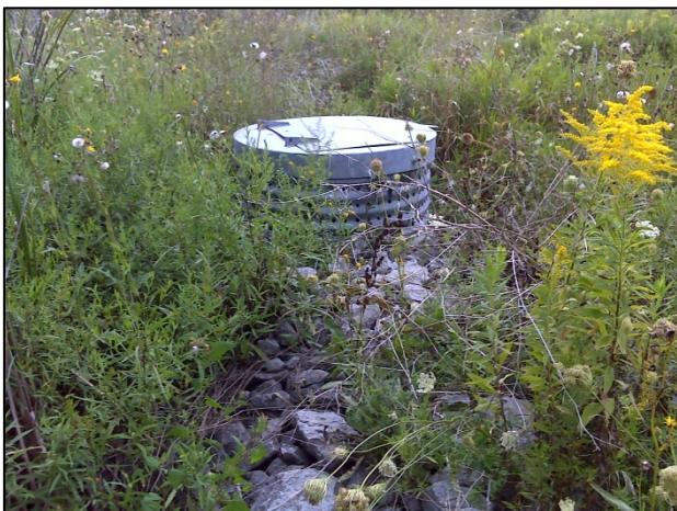
R7a: Hickenbottom inlet located a short distance west of previous photo (Summer 2015).
