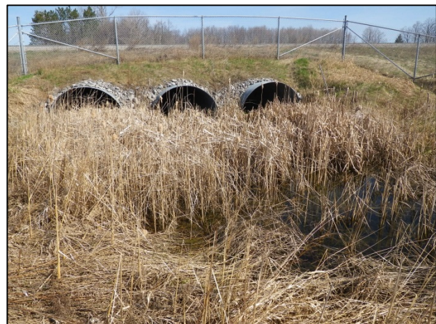
D11: Facing north (upstream) from the runningway (Spring 2015).
